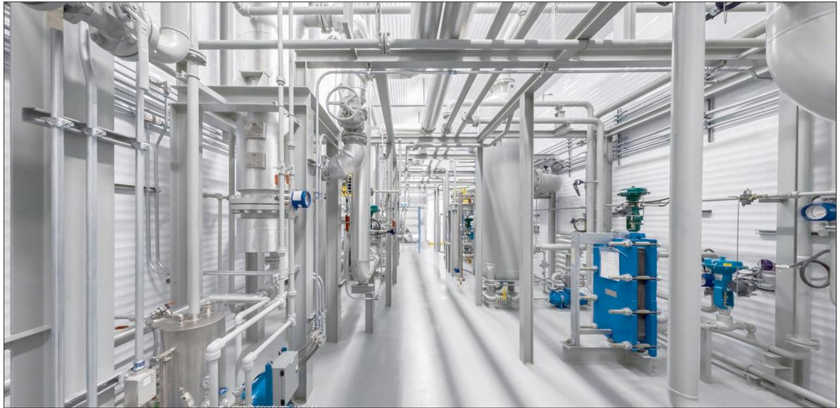
*Delta's modularly designed, commercially ready, CO<sub>2</sub> capture unit*
