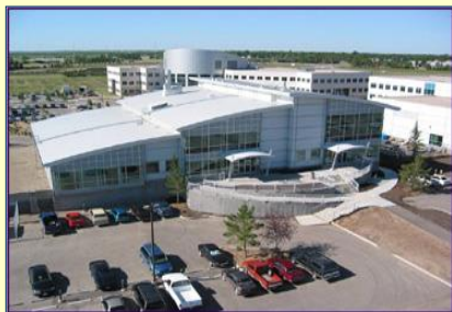
International Test Center for CO2 Capture - Home of HTC's Technical Services Center
